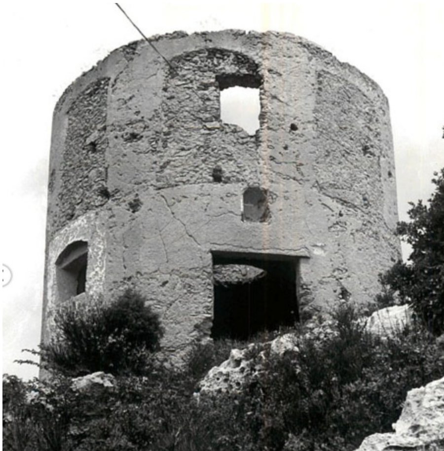
The Verezzi tower, before being closed and modified, in the eighties.
