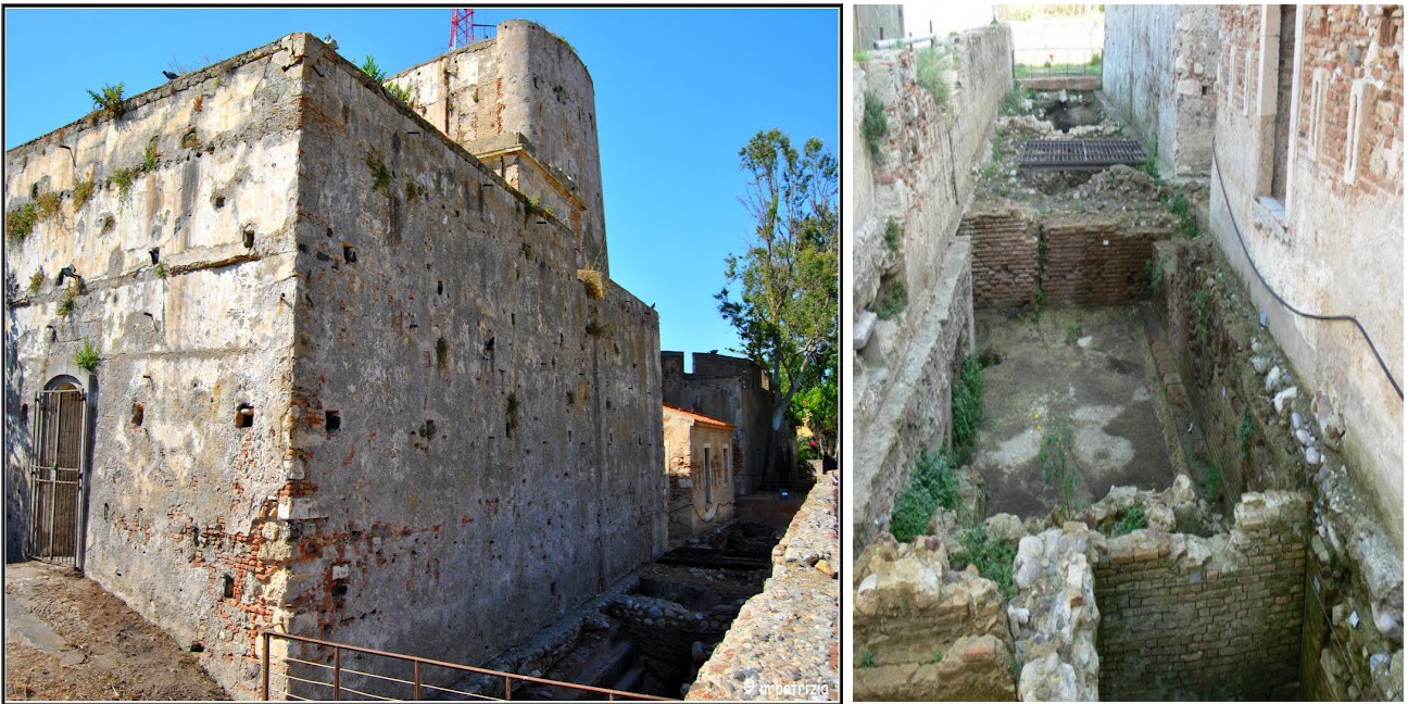
Capo Peloro Roman lighthouse excavations, under the “English Fort”, definitely more attractive than today's beacon
