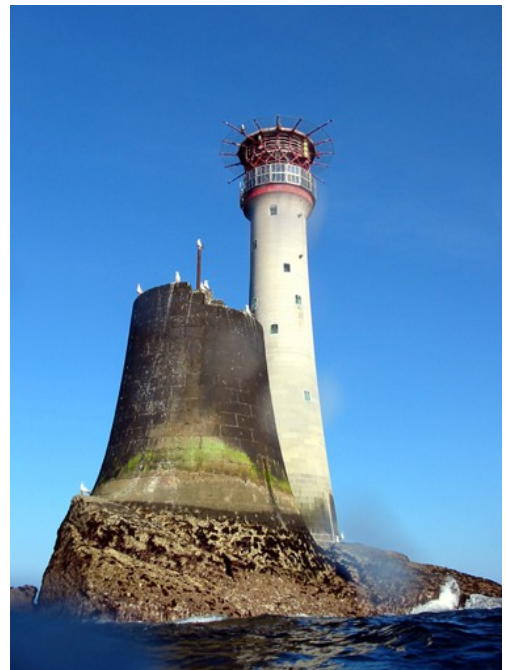
Evolution of increasingly resistant towers at Eddystone rock, the last has its own large foundations, no longer lies on the rock
