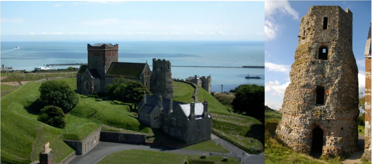
Dover Roman Lighthouse, 1 st century AD
